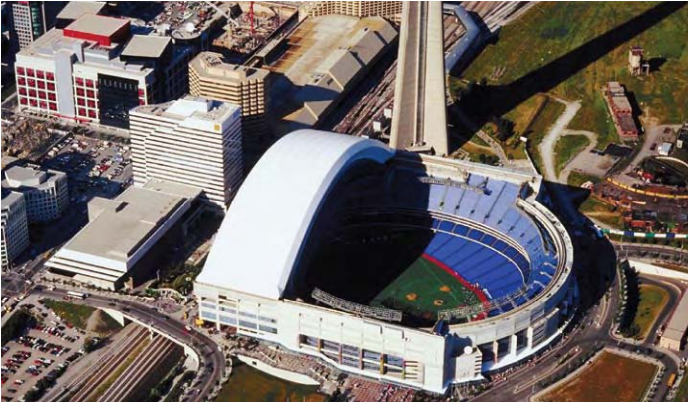
Fig. 7 The Toronto Blue Jays Stadium uses Timken bearings in the moveable stadium roof
