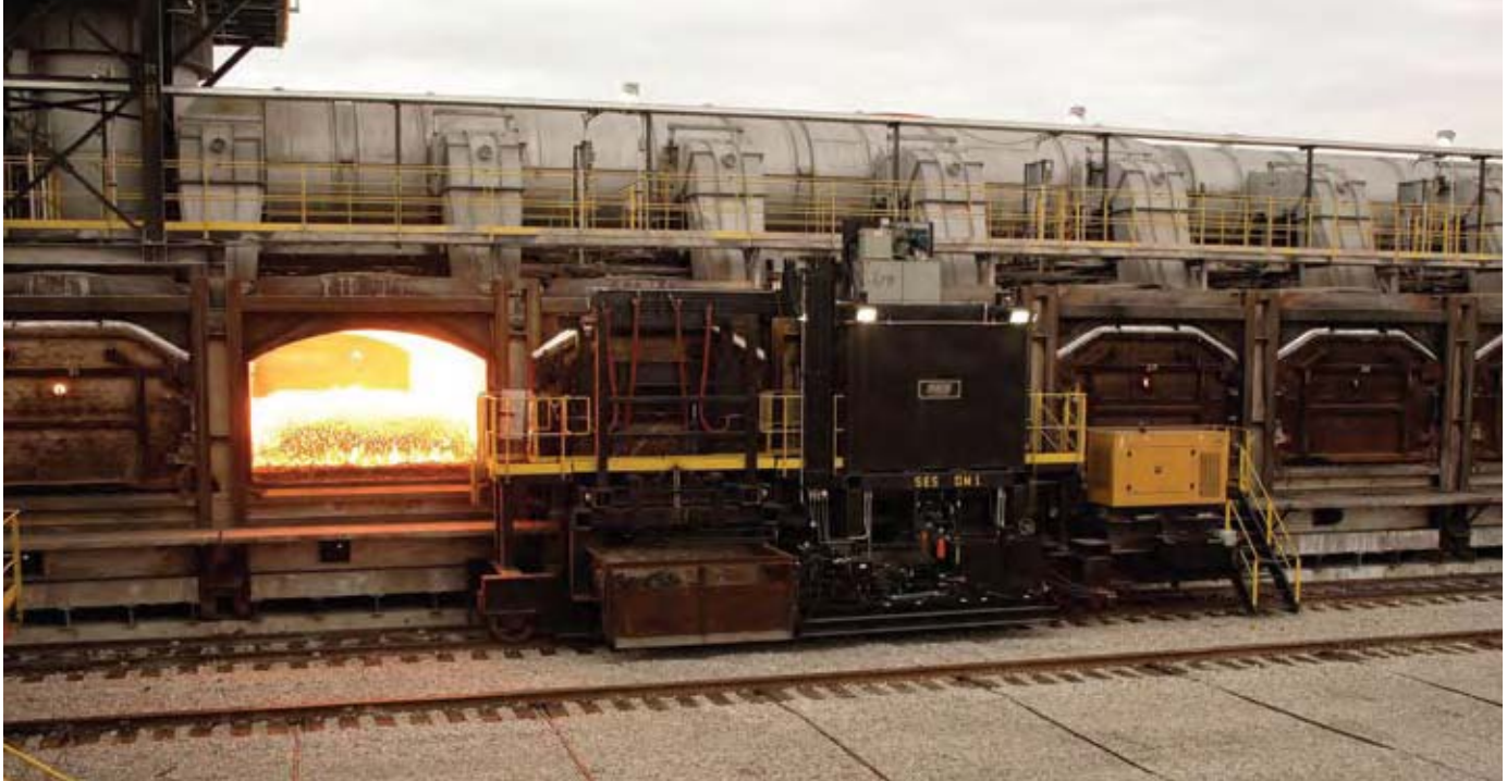
Fig. 20 Coke transfer car equipped with AP bearings
